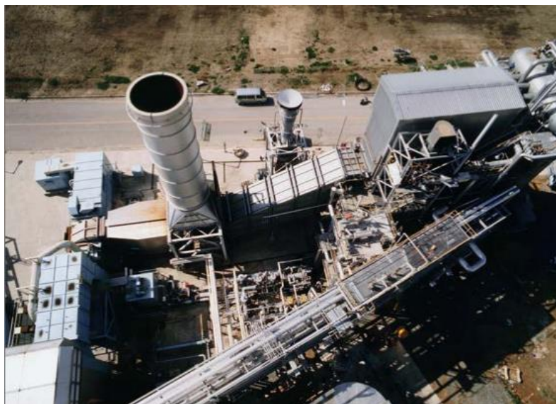
Figure 1 - 6B.03 gas turbine currently burning ~ 70%-vol hydrogen in a refinery in South Korea
